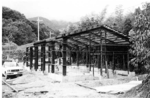
▶着々と進む尾上原資材保管施設
